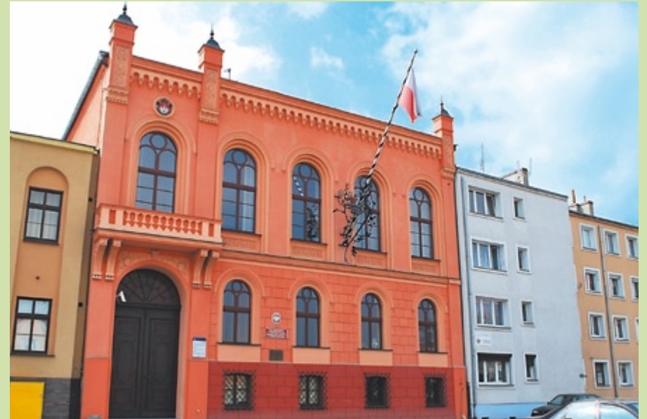
The former Town Hall
